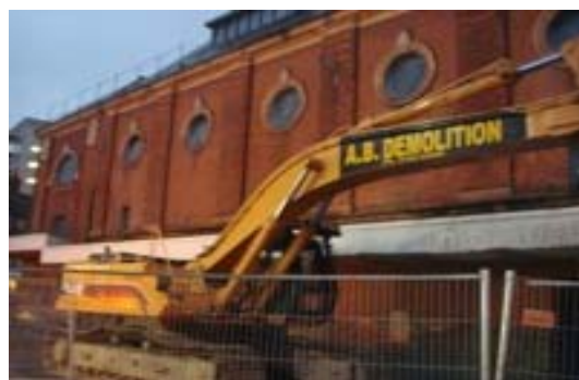
DEMOLITION OF ROOF AND WALLS
